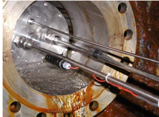
Installation of first model canister assembly
